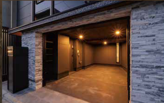
Facade / Built-in Garage
